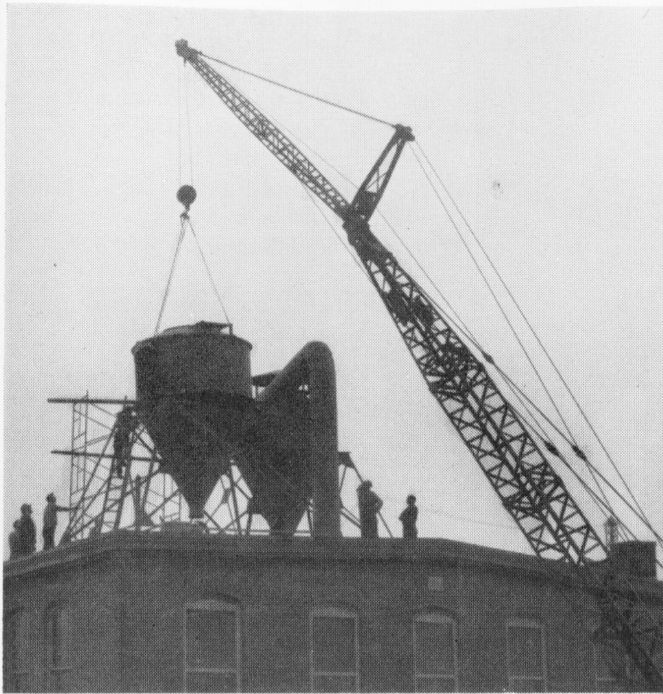
Bldg. #54, five stories tall, is dwarfed by the 100-ft. boom of the crane which holds the drum of a dust collector suspended high over Mill Street. The drum, raised from the roof of Bldg. 54, is being carried over the street, to be set down on a trailer truck in the parking lot.
