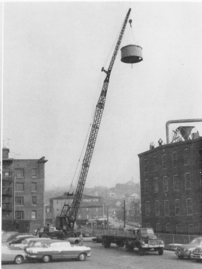
Bldg. #54, five stories tall, is dwarfed by the 100-ft. boom of the crane which holds the drum of a dust collector suspended high over Mill Street. The drum, raised from the roof of Bldg. 54, is being carried over the street, to be set down on a trailer truck in the parking lot.
